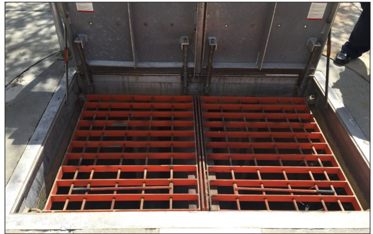
Figure 6. Current pump station with safety grate.
