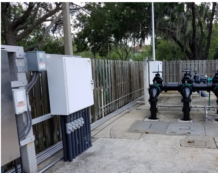
Figure 1. Existing station tie-off to electrical panel supports.
