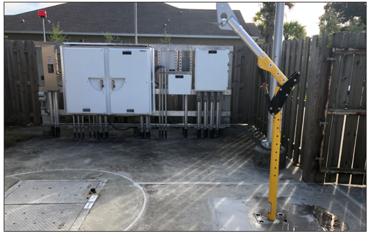
Figure 17. Recently installed pedestal mount anchor.
