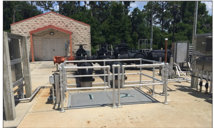
Figure 4. Existing site with permanent railing.
