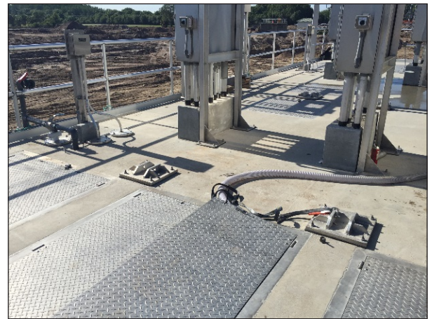
Figure 8. Fall arrest anchor post (left) and post ground anchors (right).
